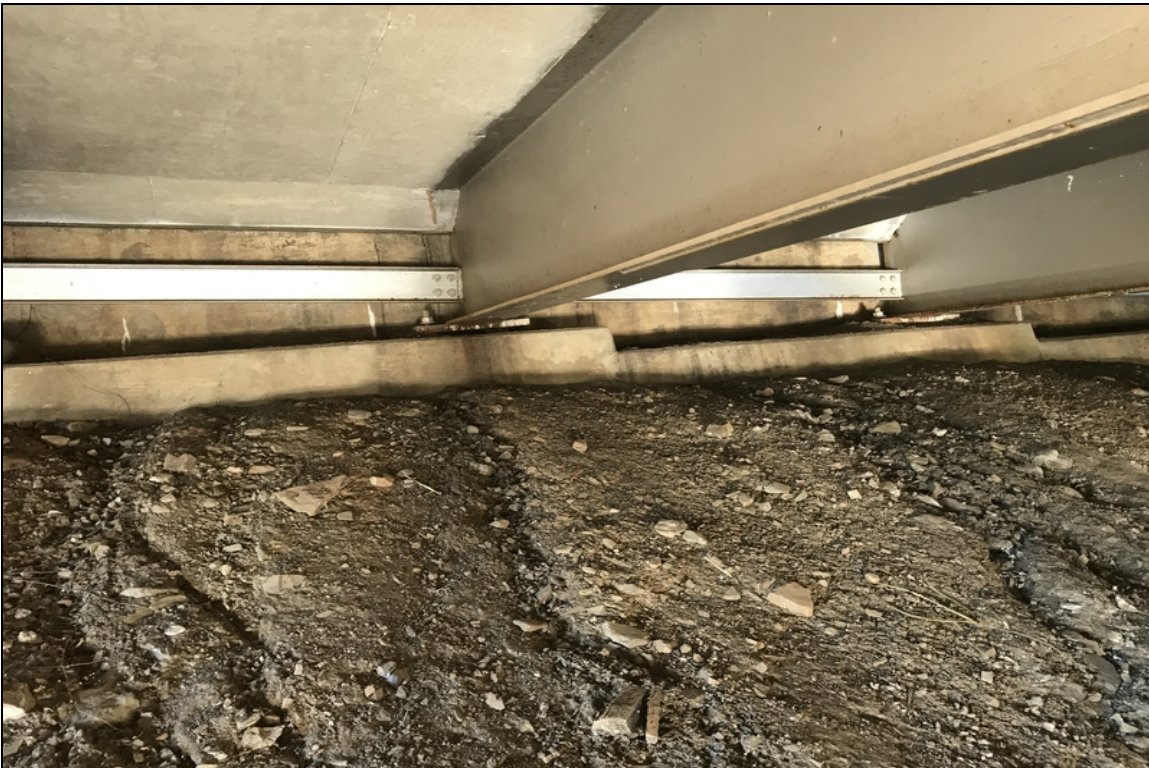
Bent 1 abutment has cracks with efflorescence in the back wall.
