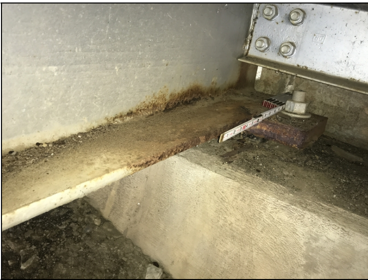
Girder 3 bent 1 has pitting up to 1/16" to bottom flange.
