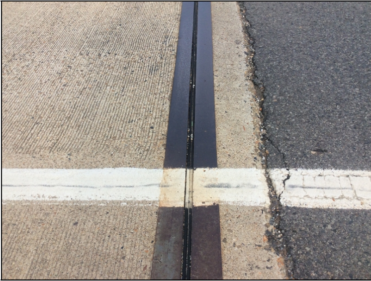
Bent 5 right side, joint has lost adhesion and is leaking.
