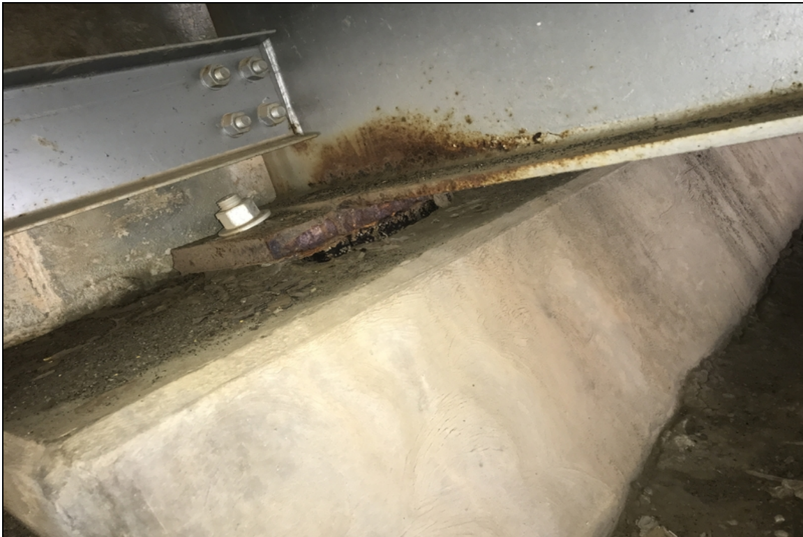
Bent 5 beam 5 sole plate has active corrosion.
