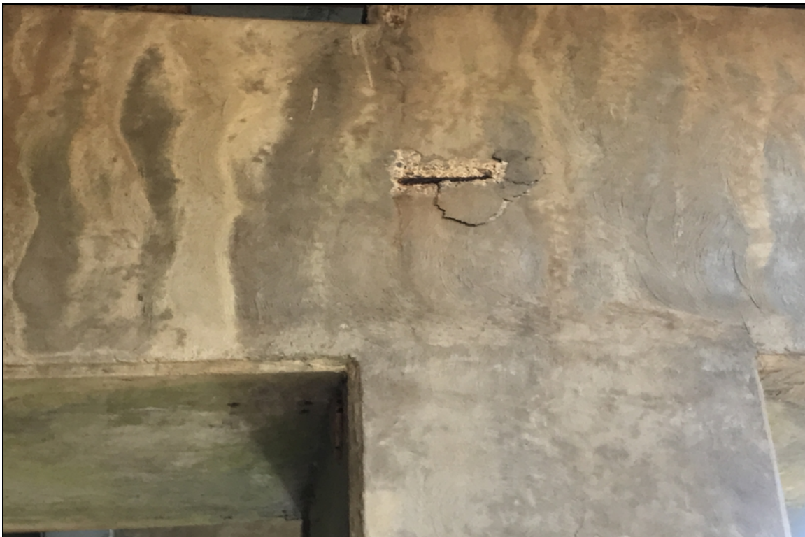
Bent 2 cap back has spall with exposed rebar.
