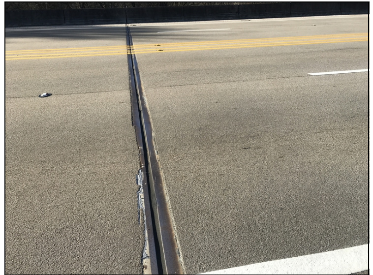
Joint seal at bent 4 has been repaired.
