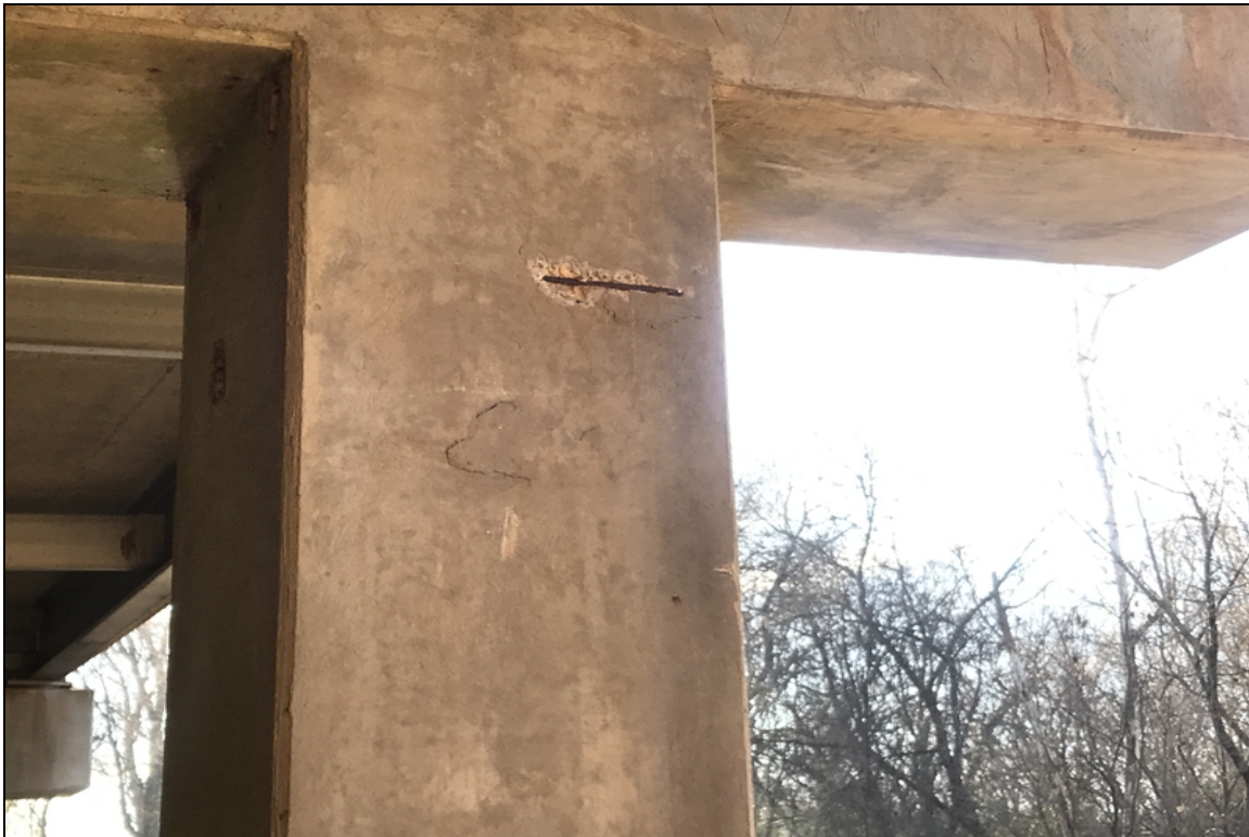
Bent 2 column 4 has spall with exposed rebar.
