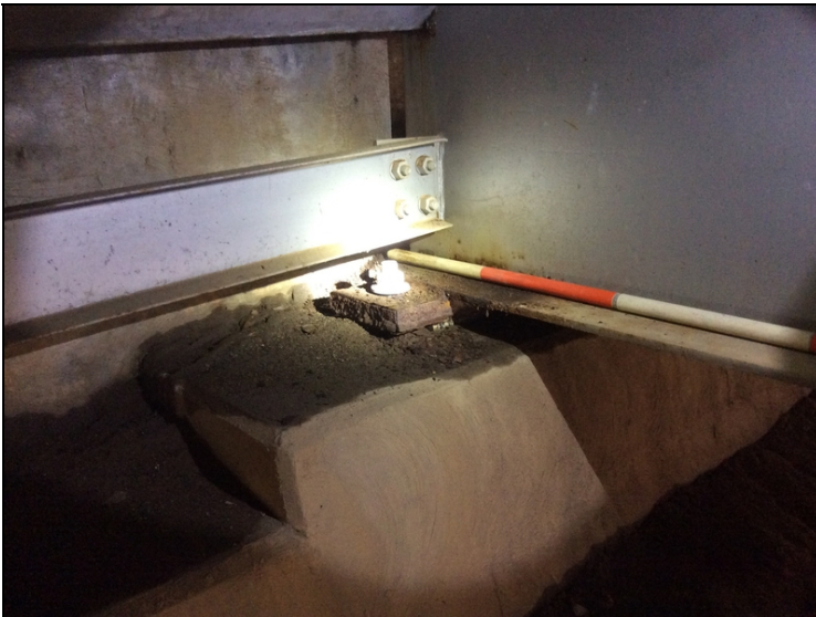
Bt. 4, Bm. 7, corrosion & minor pitting on the bottom flange & sole plate of bearing.
