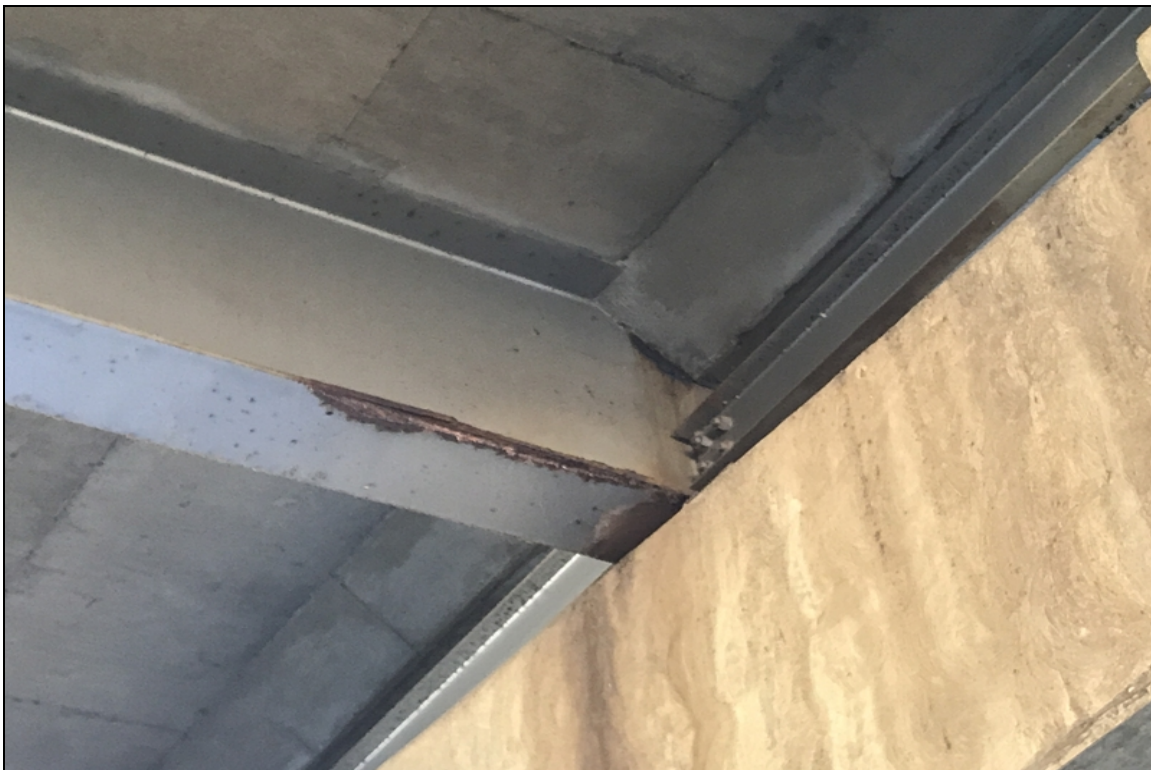
Bent 2 beam 3 has corrosion lower flange and upper web haunch area.
