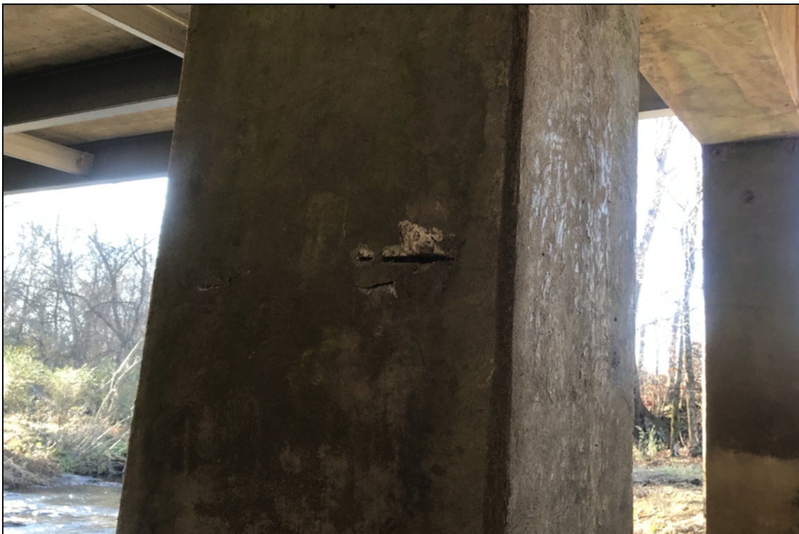
Bent 2 column 3 left side has spall with exposed rebar.
