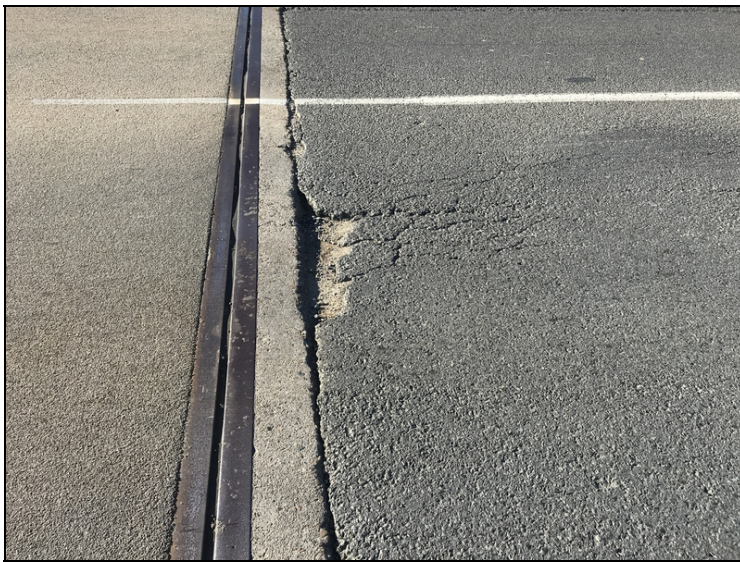
Pothole in asphalt approach at West end of bridge.
