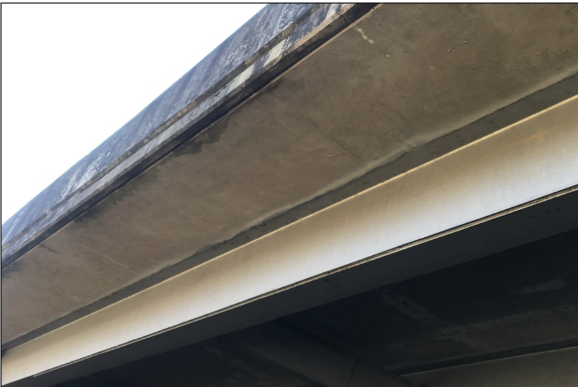
Span 3 left side soffit overhang has cracks with efflorescence.
