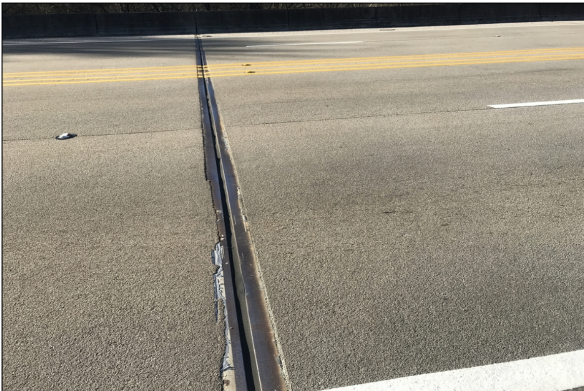
Joint seal at bent 4 has been repaired.
