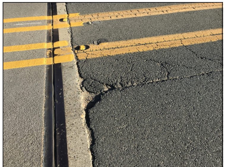
Pothole in asphalt approach at East end of bridge.
