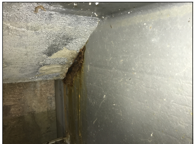
Bent 1 girder 4 right side has pitting up to 1/8" in the haunch area of the upper web.
