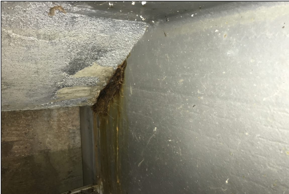
Bent 1 girder 4 right side has pitting up to 1/8" in the haunch area of the upper web.
