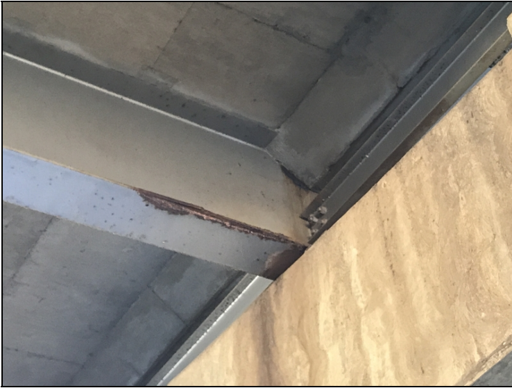
Bent 2 beam 3 has corrosion lower flange and upper web haunch area.
