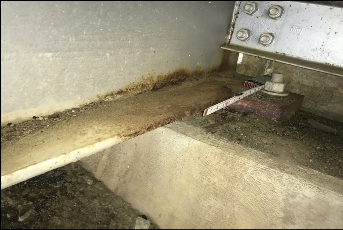
Girder 3 bent 1 has pitting up to 1/16" to bottom flange.
