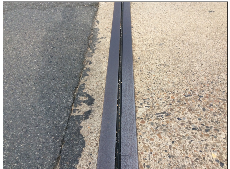
Bent 1 joint has lost adhesion and is leaking.
