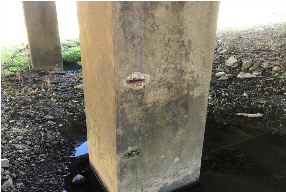
Bent 3 column 2 has spall with exposed rebar.
